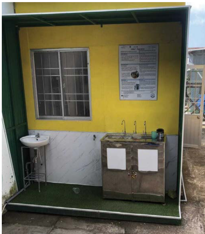
Fig. 1: Service water is distributed via the house network and can be taken from the outside water tap, while drinking water is only provided in small quantities when required at the stainless steel sink outside the operating building
