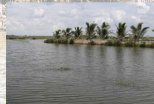
Salinity protection gate
